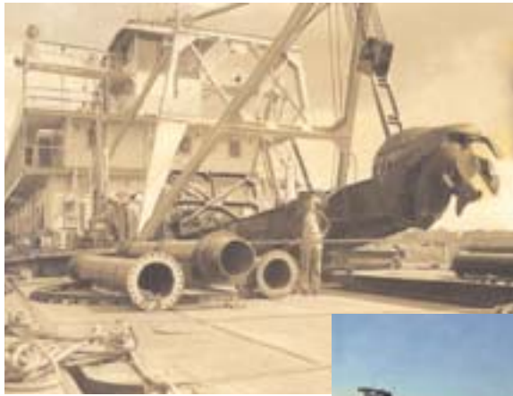
The cutterhead carves out dredge spoils that are then sent through hundreds of feet of pipes. (Winona Country Historical Society)
