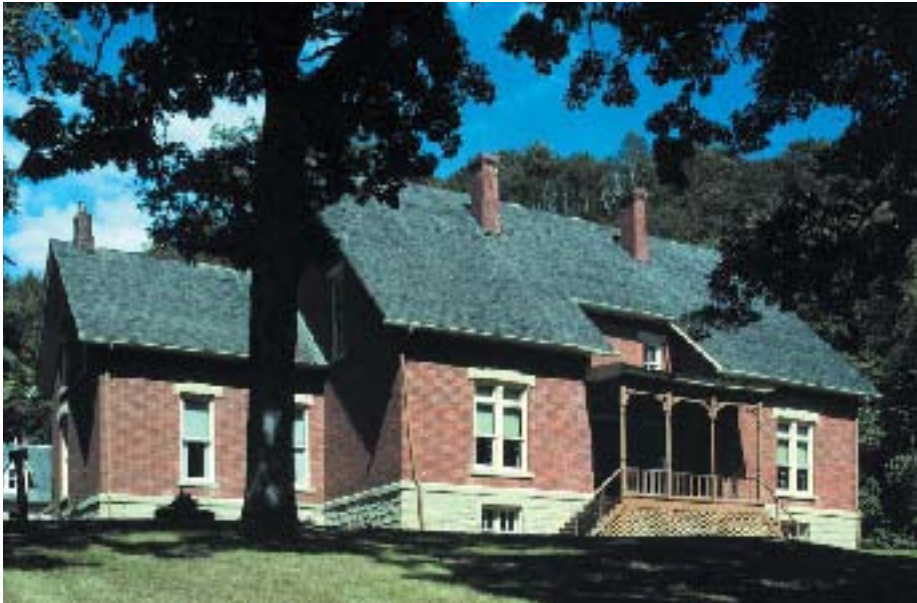
This summer residence on the grounds of Stonefield Village was built in 1893. Some of the outbuildings remain from governor Nelson Dewey's earlier residence. (Stonefield Village)
